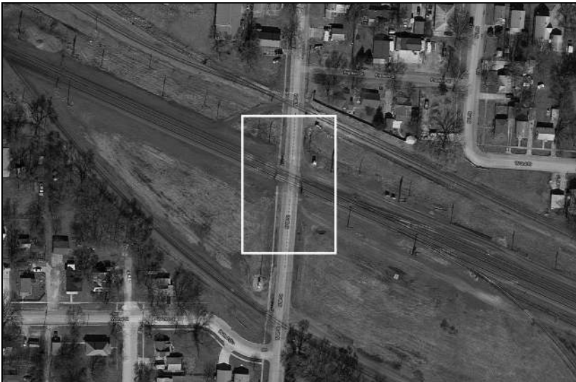
Figure 2: HRGC at the M Street Crossing in Fremont, Nebraska
