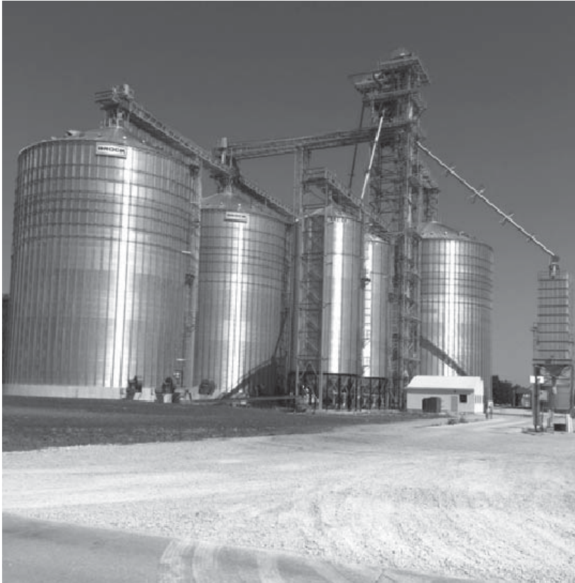
Figure 1: New Addition to Elevator Located on an Abandoned Rail Line at Luther, Iowa, 2016
